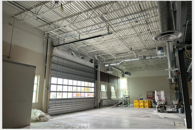
A look into the Skills Lab Addition where wall and ceiling painting has begun with finished MEPF rough-ins in place.
