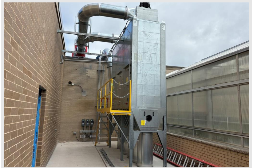
The new dust collector unit outside of the Skills Lab Addition and Wood Shop is in place and being prepared for startup!
